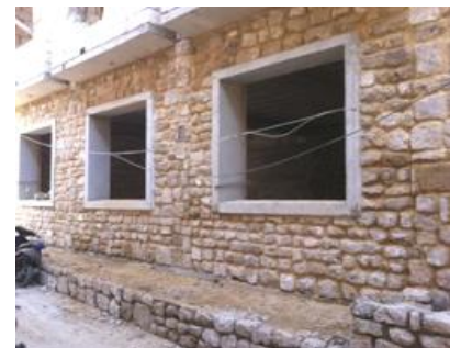
Figure 17- new building in the old city using the old material from demolished building to produce a contemporary design proportions (photo taken by researcher, 2014)
